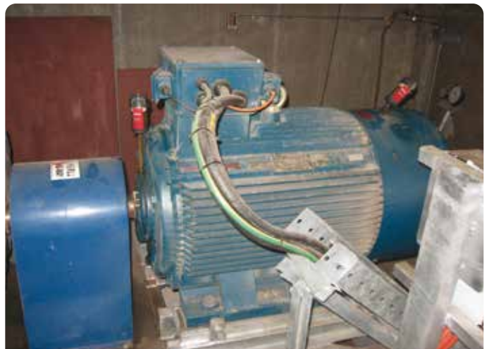
Application Electric motor Lubricator perma NOVA130 Installation kit Direct mount
