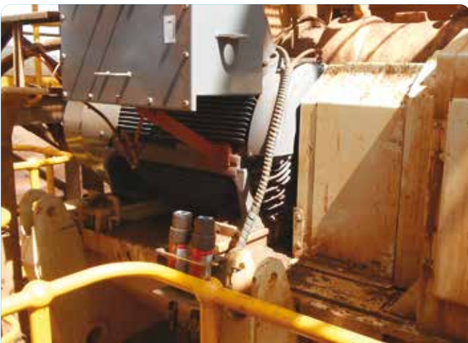
Application Electric motor Lubricator perma STAR VARIO L250 Installation kit K230C
