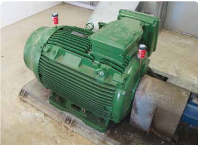
Application Electric motor Lubricator perma FLEX125 Installation kit Direct mount
